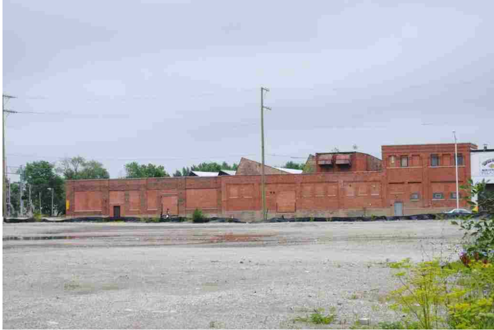
Figure 4.6 - Contemporary Photograph - Former Norton Brothers Can Works Site. The American Can Company plant was demolished in the late 1990s. The only remaining original structure from the Norton Brothers Can Company is the Tin Mill with the "saw tooth roof" in the background. Photograph taken by the author looking east, July 2013.
